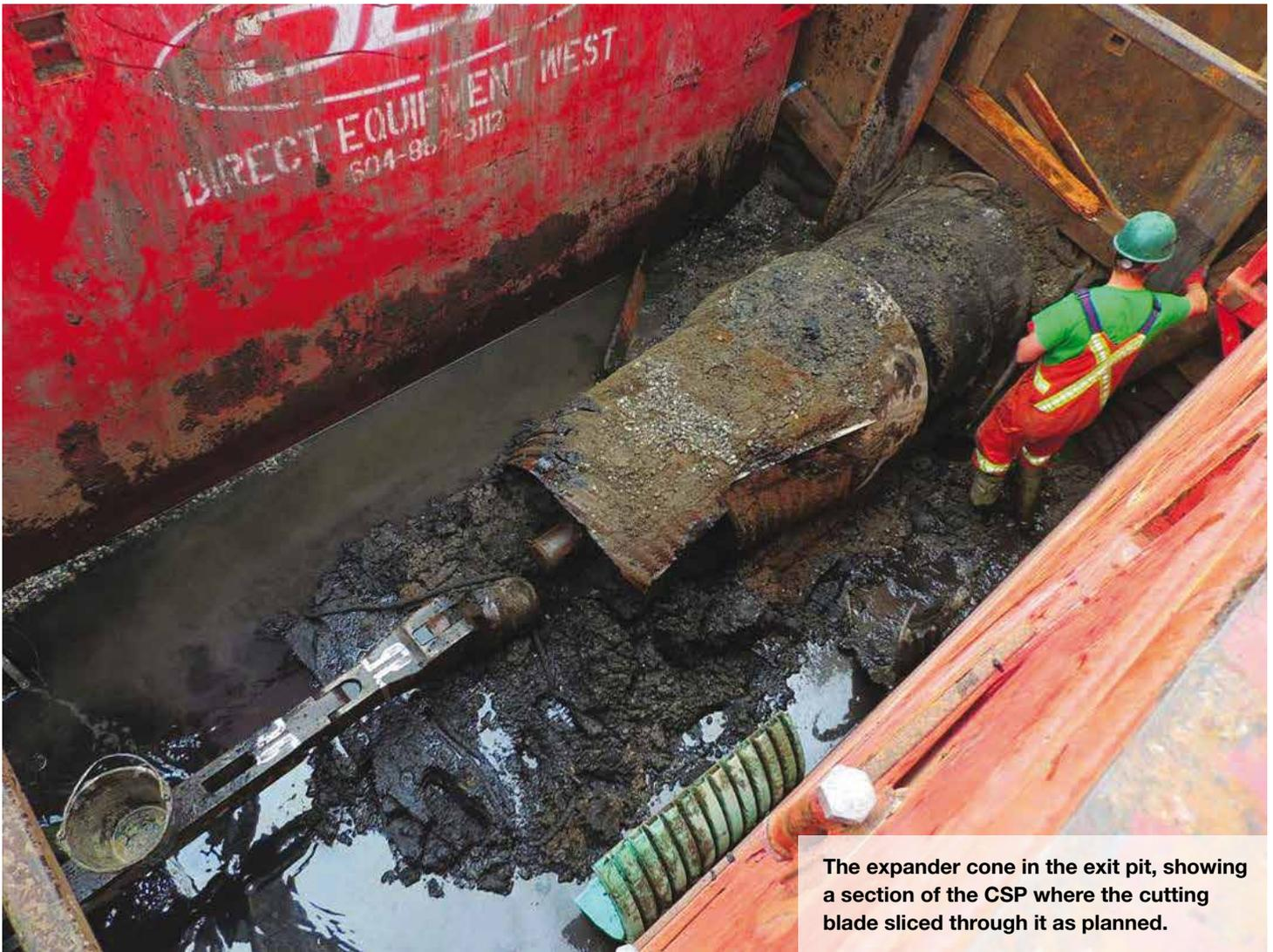
The expander cone in the exit pit, showing a section of the CSP where the cutting blade sliced through it as planned.
