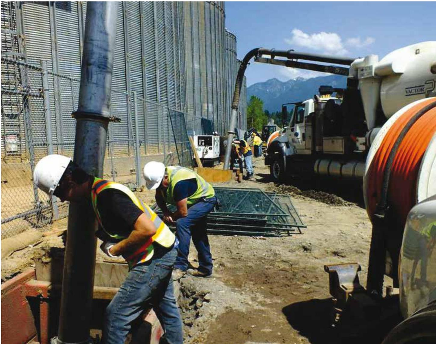
Deacon said the job was a challenge for PW Trenchless Construction due to the relatively large 42-inch pipe needed for the catchment area, and the pipe bursting equipment it required.
